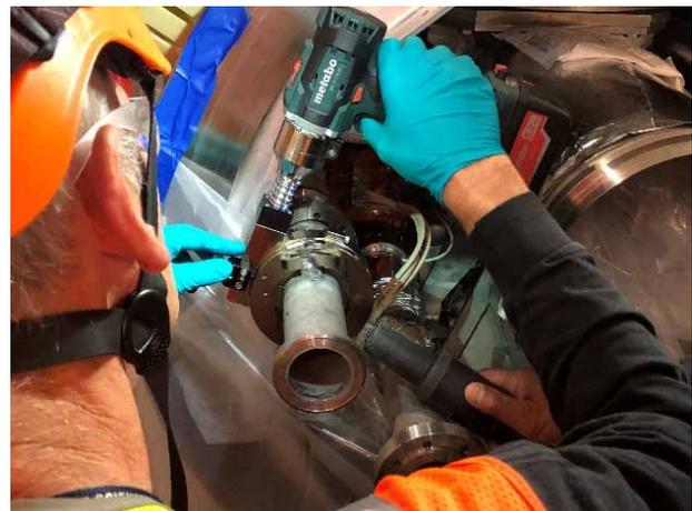
Figure 3: Cutting helium process pipes to length.
