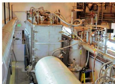
Figure 2: A-Tank cryostat in ATLAS beamline.
