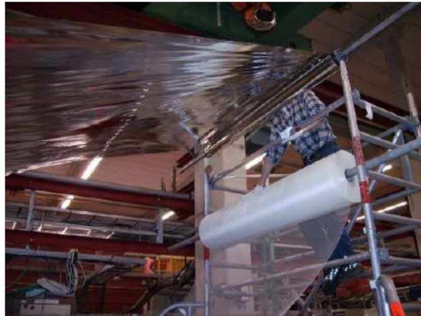
Figure 61: Two layers of super insulation on cold mass
