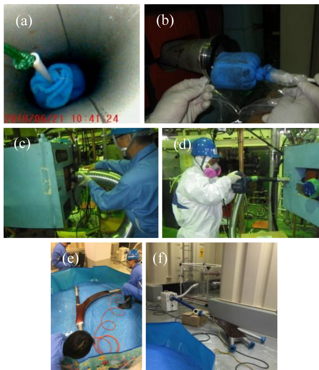
Figure 11: Pictures of cleanings of ducts and chambers in the HEBT; alcohol wiping (a,b), air blowing (c), and vacuuming (d). Two bending magnet chambers were rinsed with pressurized ultra-pure water (e,f).
