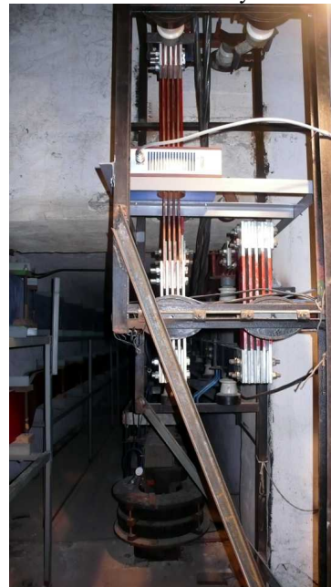
Figure 2: Current transformer ITZ Ultrastab at the current line.
