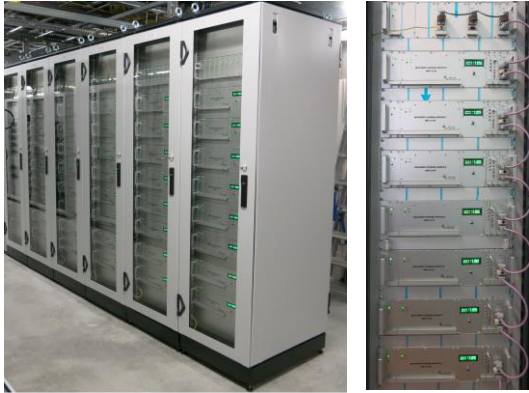
Figure 5: Racks with power supplies: with redundancy system at XFEL (left) and the burn in rack with the measurements crate (right).
