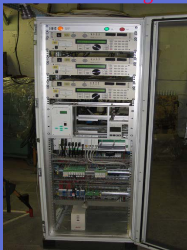
Power supply and control system of SC magnet
