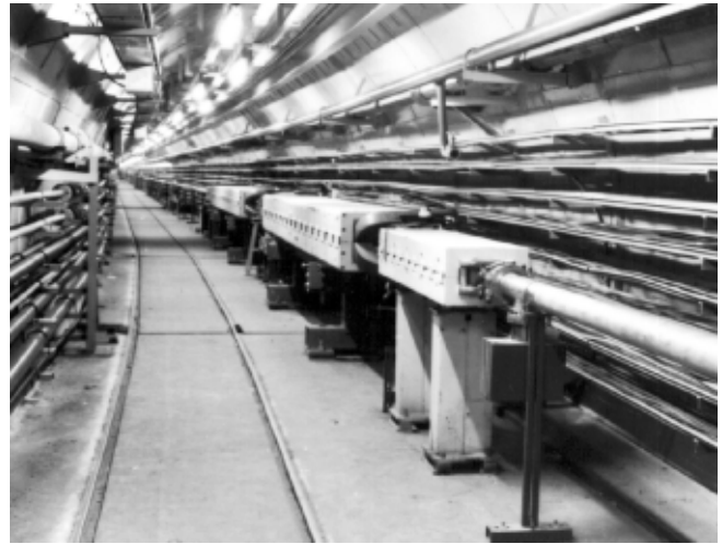
Figure 4: Beam transfer line tunnel.
