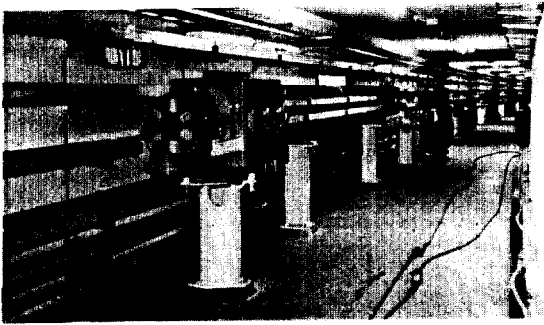
Fig. 2 Magnet assembly in the tunnel
