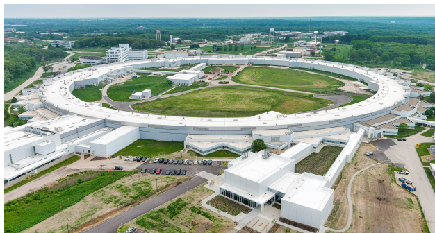
Figure 1: New Long Beamline Building (LBB).
