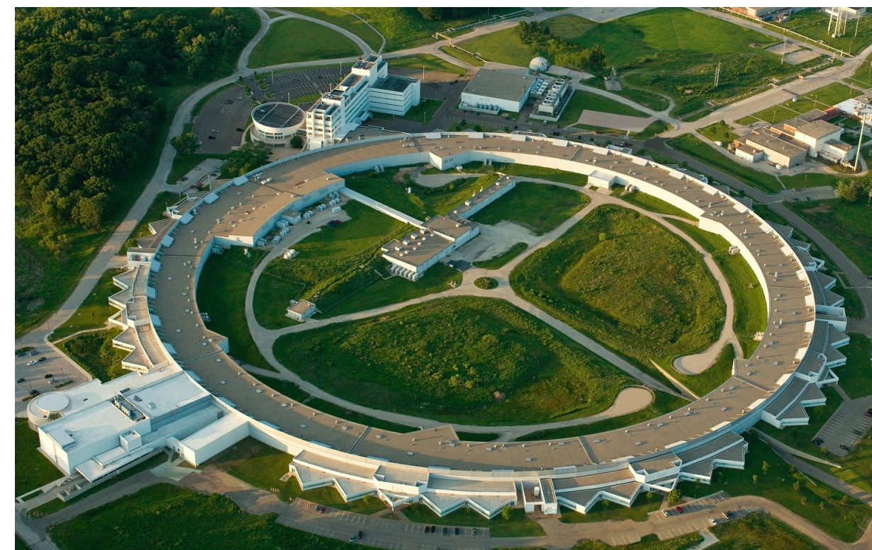
Advanced Photon Source at Argonne National Laboratory, Lemont, IL USA
