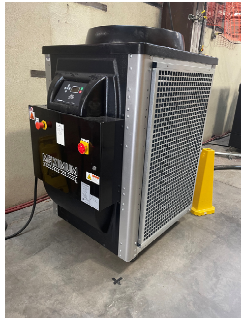
Figure 1: Photograph of the CARIE klystron (top); photograph of the chiller that supplies cooling water to the klystron and the facility (bottom).
