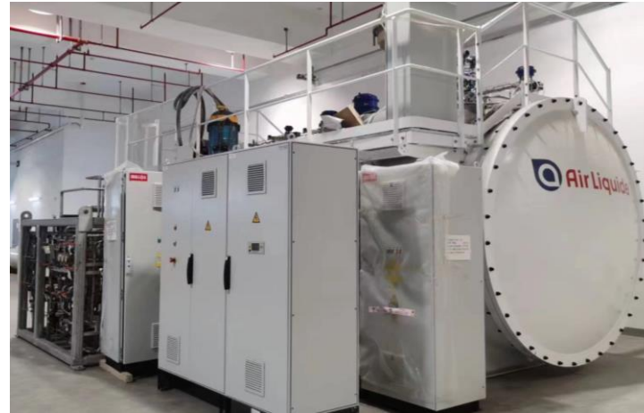
2K cold boxes (X2) & Distribution box (X3) in commissioning
