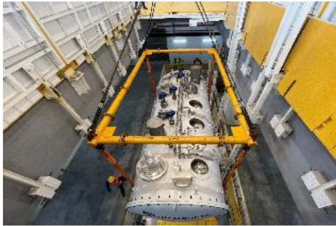
2K cold boxes (X2) & Distribution box (X3) in commissioning
