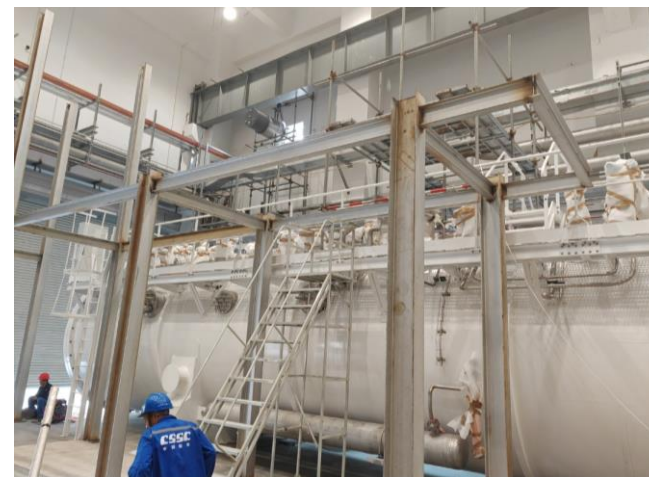
2 nd 4.5K cold box installed
