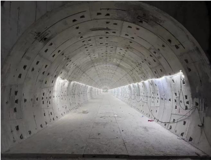
Eastern tunnel between Shaft #3 and Shaft #4
