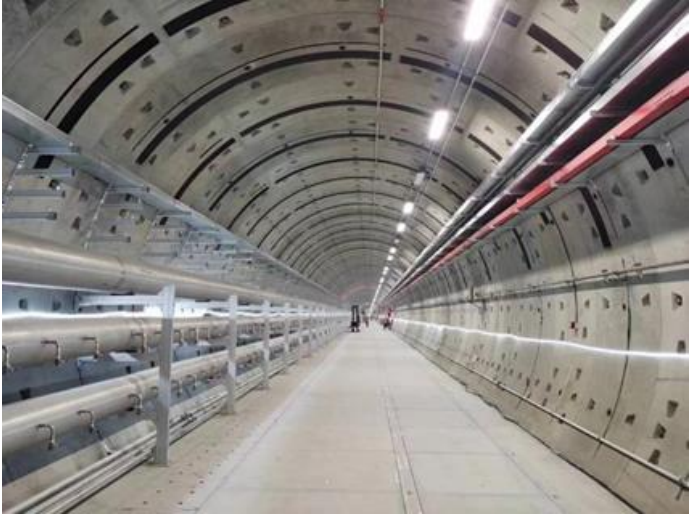
Tunnel between Shaft#1 and Shaft #2
