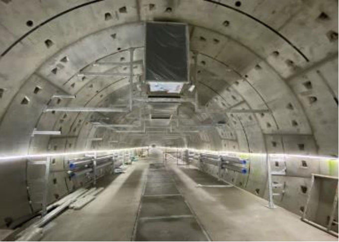
Eastern tunnel between Shaft #2 and Shaft #3
