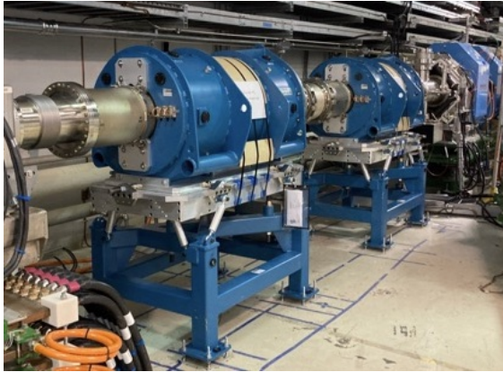
Figure 2: Solenoids installed in the SNS ring.
