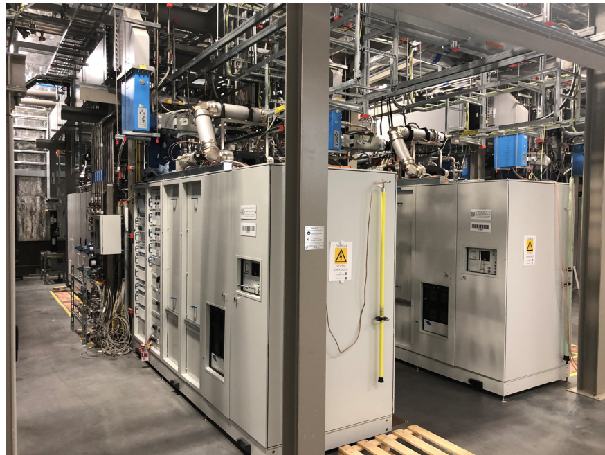
Klystrons based RF stations in Elliptical Section Modulators designed at ESS and provide in kind from ESS-BL
