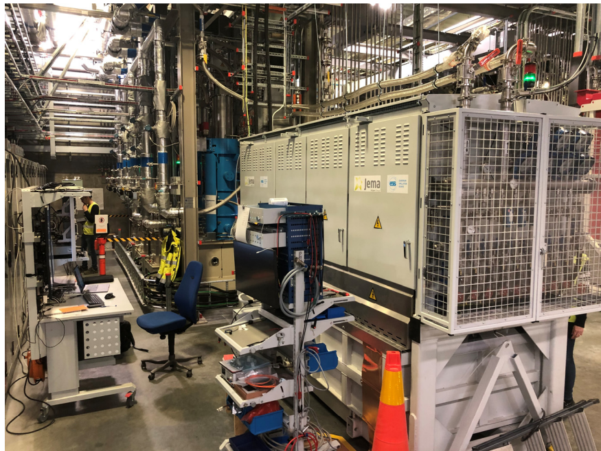
Tetrode RF Power stations in Spoke Section Tetrode RFPs provided in kind from Elettra
