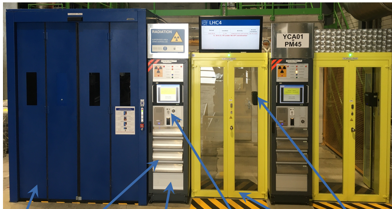
MAD Safety token distributors Instrument rack Intercom Badge reader Touch panel PAD Iris reader
