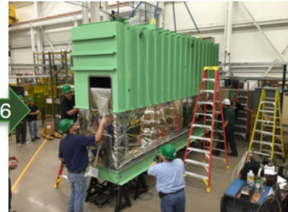
Vessel cover installation
