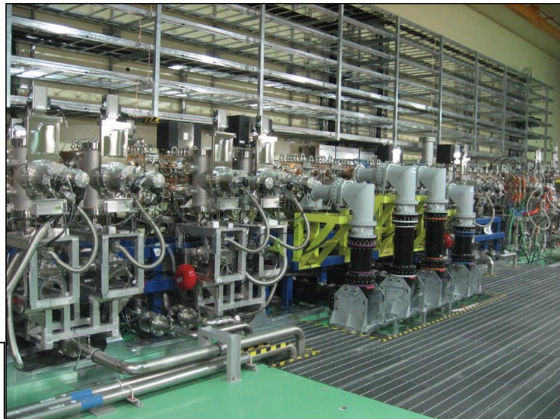
Vacuum system installation
