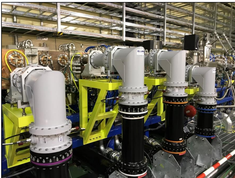
High power couplers installation
