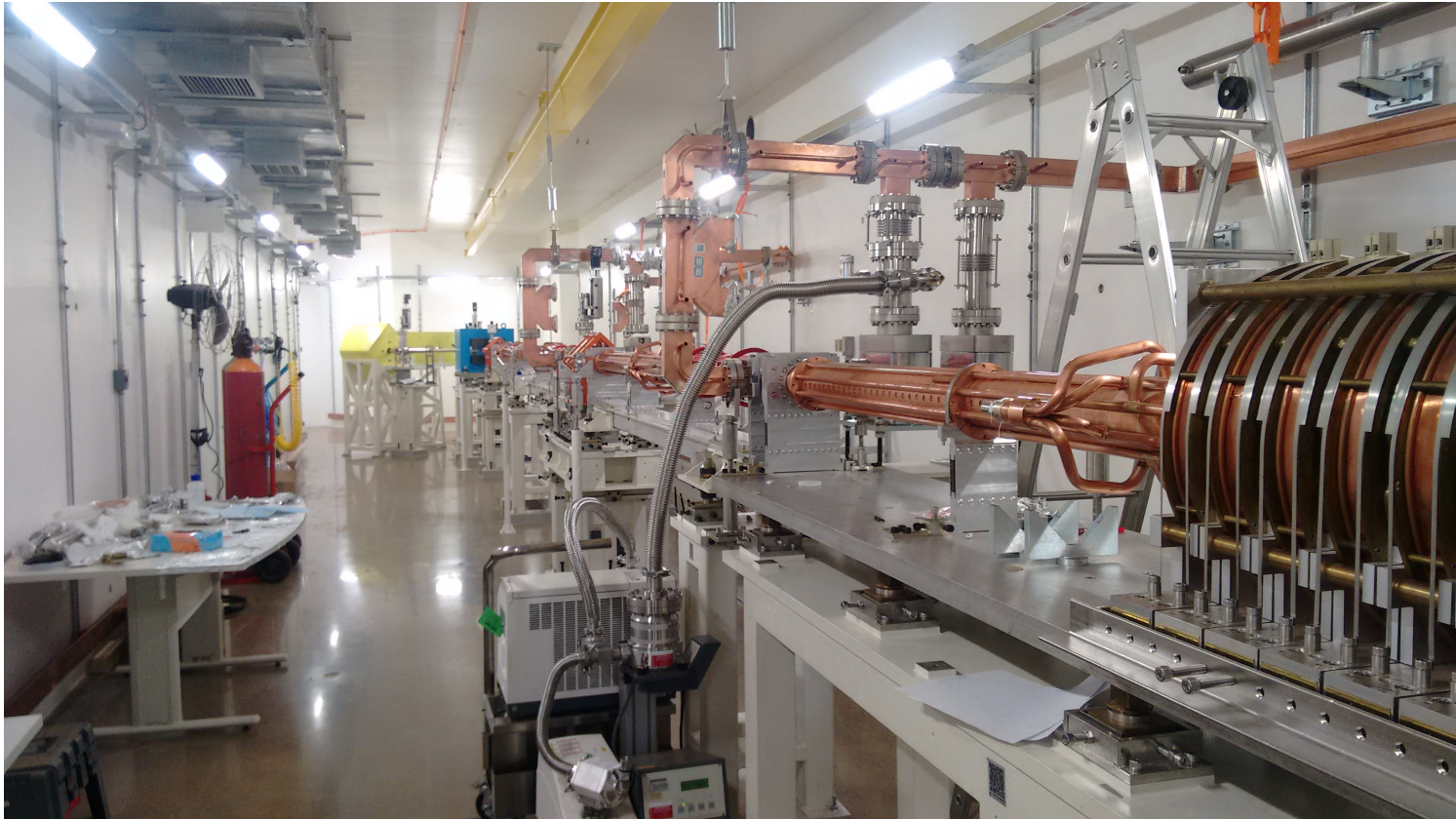
Turn-key 150 MeV LINAC bought from SINAP-Shanghai during installation
