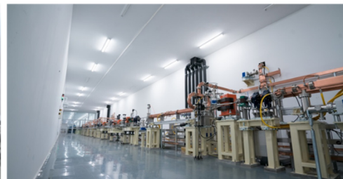
Dalian Coherent Light Source (DCLS) An EUV user facility (50 – 150 nm)
