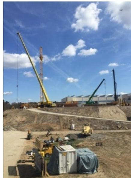
Figure 1: To enhance the radiation shielding, the soil layer on the SIS18 tunnel is presently being enhanced.
