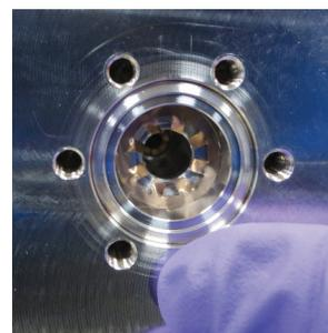
Figure 2: The recess with beryllium copper spring prior to the feedthrough installation.
