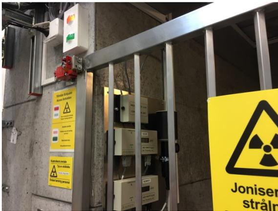
Figure 4: Bunker door showing clearing indicator lamp and the switch to trigger the PLC interlock and the hardware interlock of the RF stations. Just behind the closed door you can.
