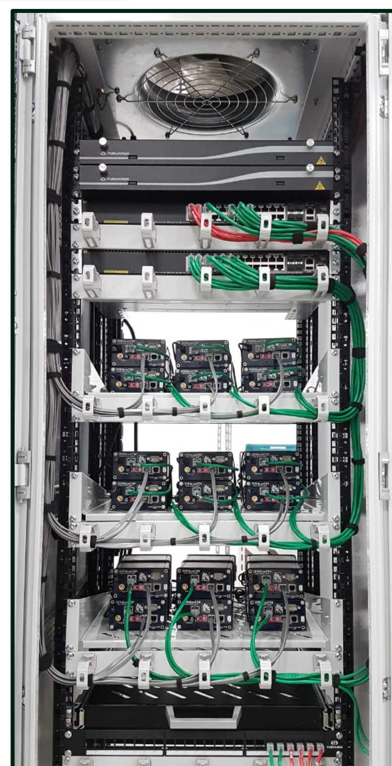
Figure 3: Controls System distributed cabinet, with Beaglebone Black as a node.
