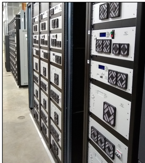
Figure 1: Modular type SCM PS.
