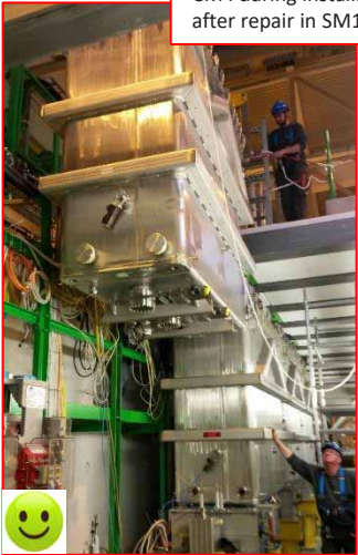
CM4 during installation after repair in SM18
