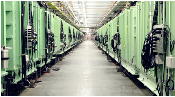
Figure 2: FRIB tunnel after the completion of installation.
