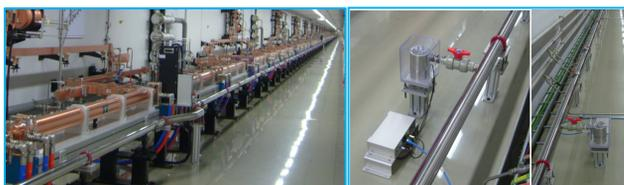
Figure 4: Condition of installed waterpipes and HLSs (Linac on the left and Undulator on the right).
