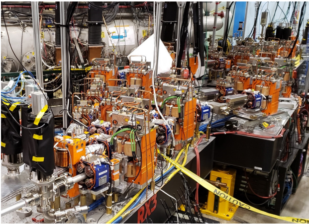
Figure 16: CBETA splitter lines, viewed from the linac end [14].
