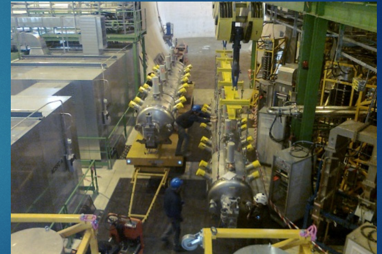
Exchange of an LHC cryomodule
