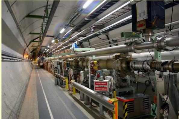
Ejected beam installed above the two circulating beams
