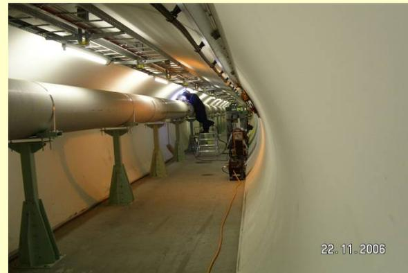
600 mm beam pipes - last 100 m before the dump absorber
