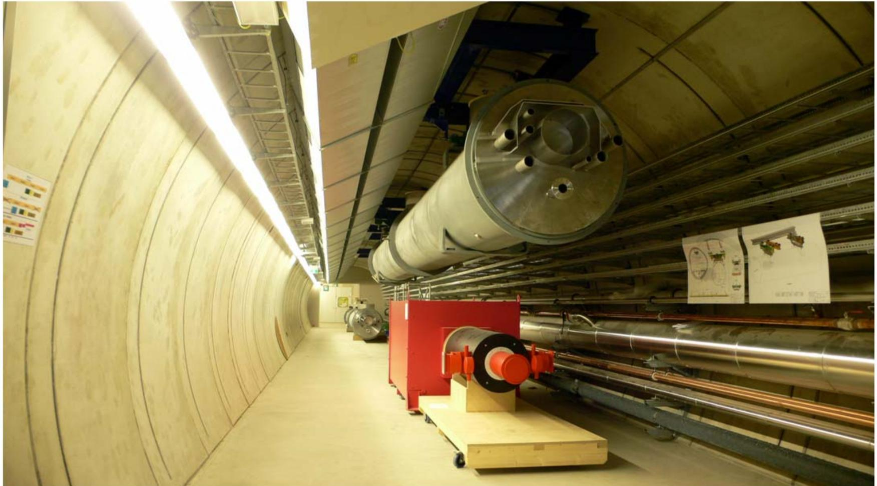
Test of installation procedures for acc. modules incl. RF
