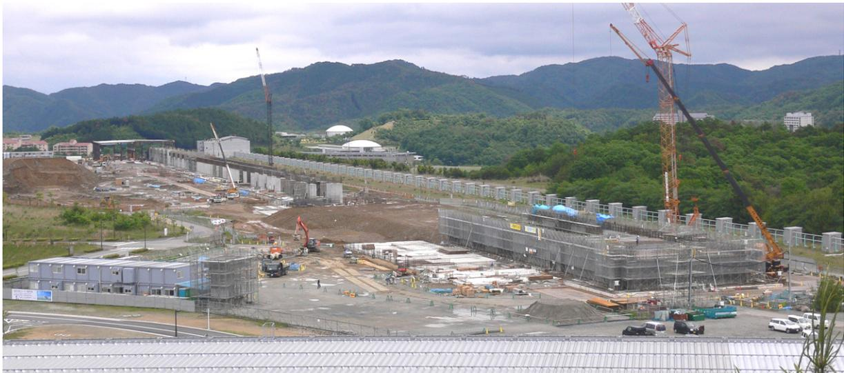
Figure 1: The XFEL construction at Spring-8 site (May 2008). The 400 m long accelerator (from left to middle), followed by the undulator hall. The construction will be completed in 2009.
