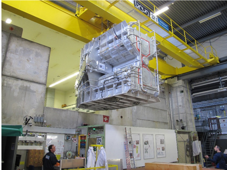
Bringing the new Resonator in the Injector 2 bunker
