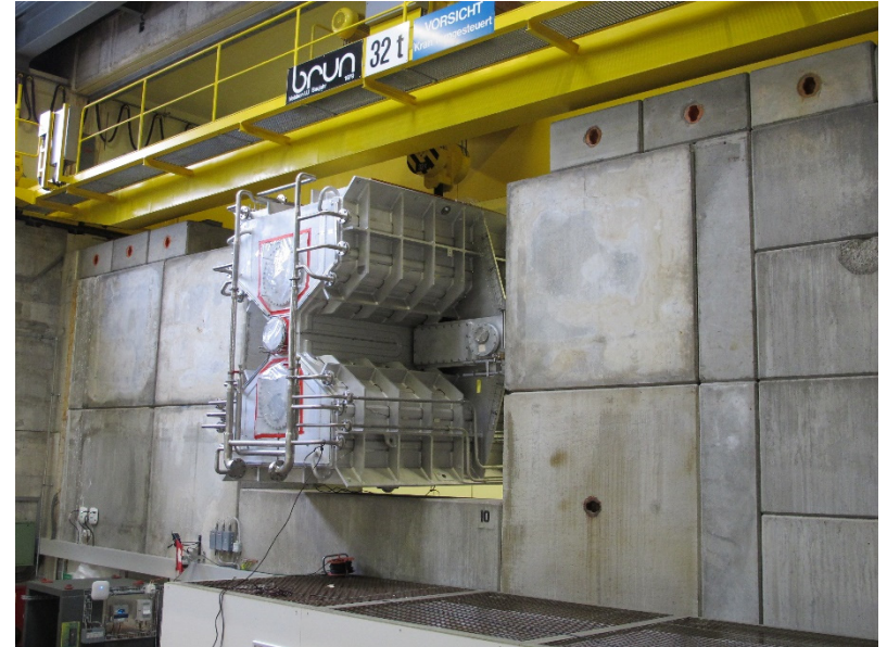
Passing trough the wall (only about 10 cm left in height)
