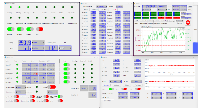
Figure 11: A control panel during the cooler commissioning.
