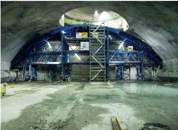
Figure 2: Vault concreting of ATLAS experimental cavern
