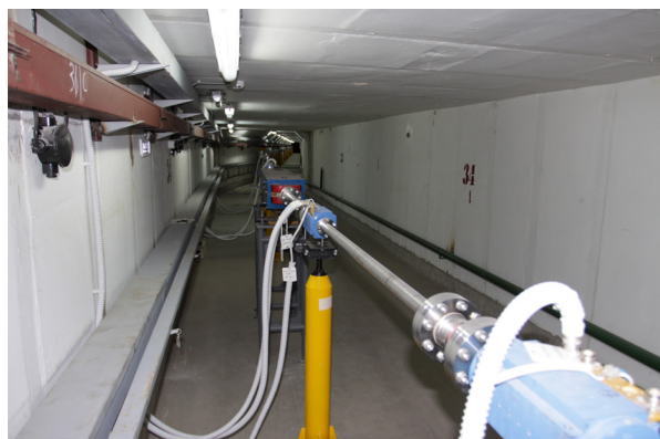
Figure 3: Transfer line K500 to VEPP-2000.
