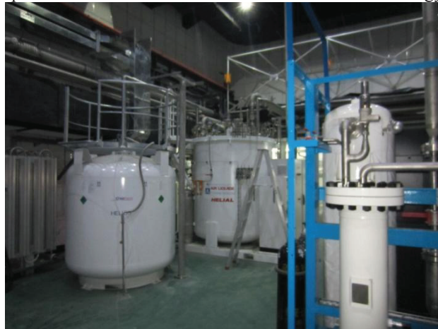
Figure 12: 2K cryogenic LHe system.
